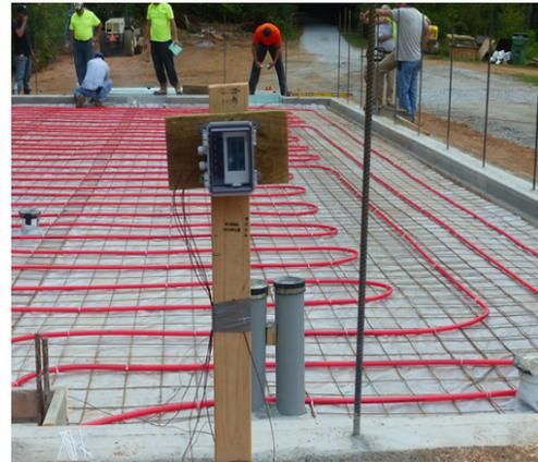
**Figure 1:** The experimental setup showing the temperature data logger and several thermocouples prior to pouring the concrete slab.
